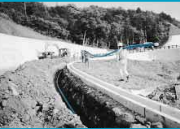
Transporting the pre-fused pipes, dimension d 90 mm, to the trench.
