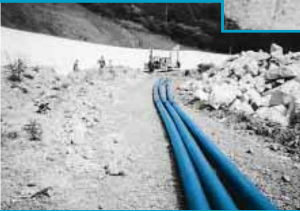
To join the 5 m long pipe sections, an ELGEF Plus socket is the answer.
