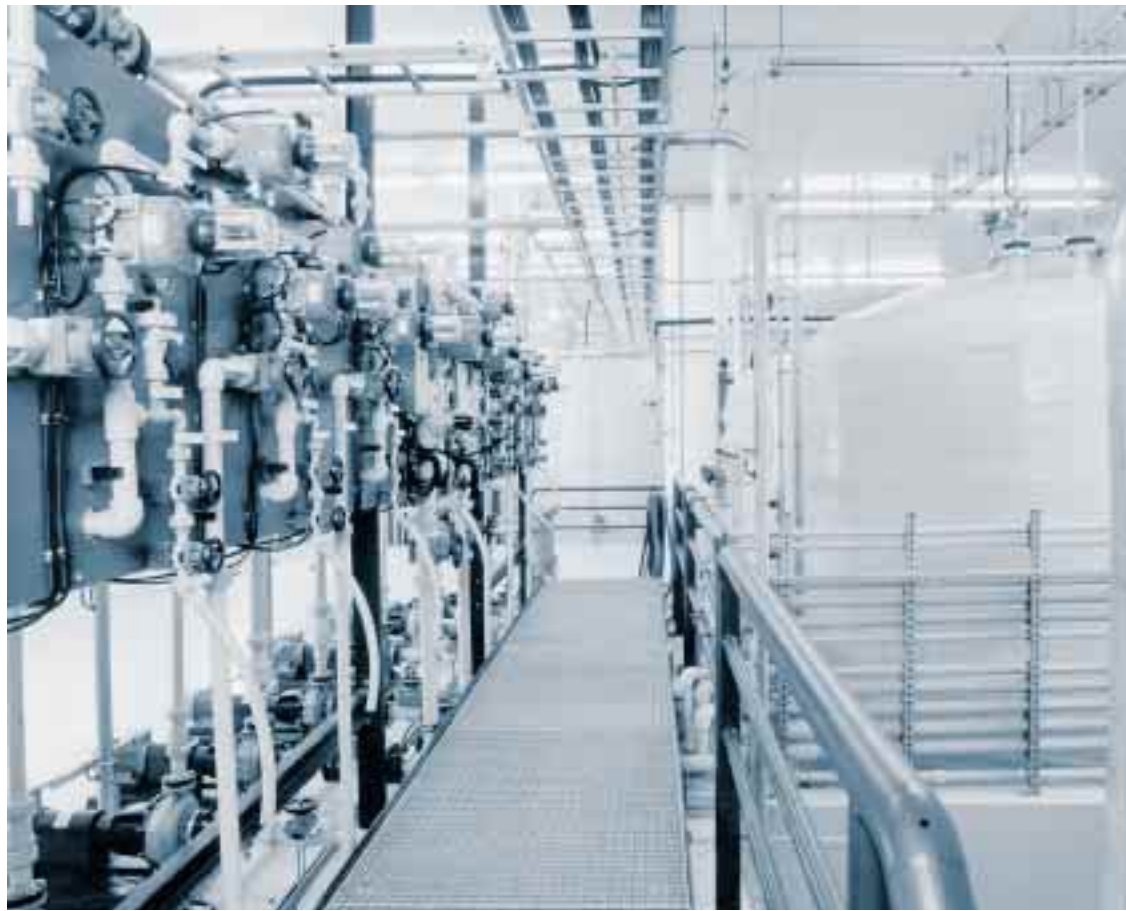
An example of a dosing plant for lyes and acids, which is made of polypropylene with pneumatic diaphragm valves.
